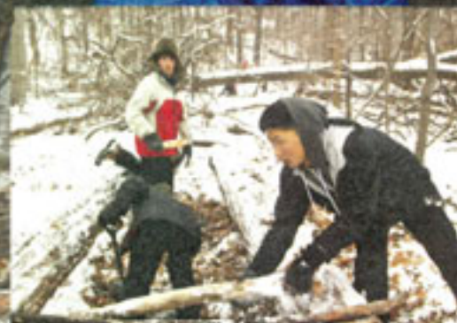
The Scouts lay down long pieces of wood to create a roof (above), before filling in the gaps with leaves and twigs (below).
